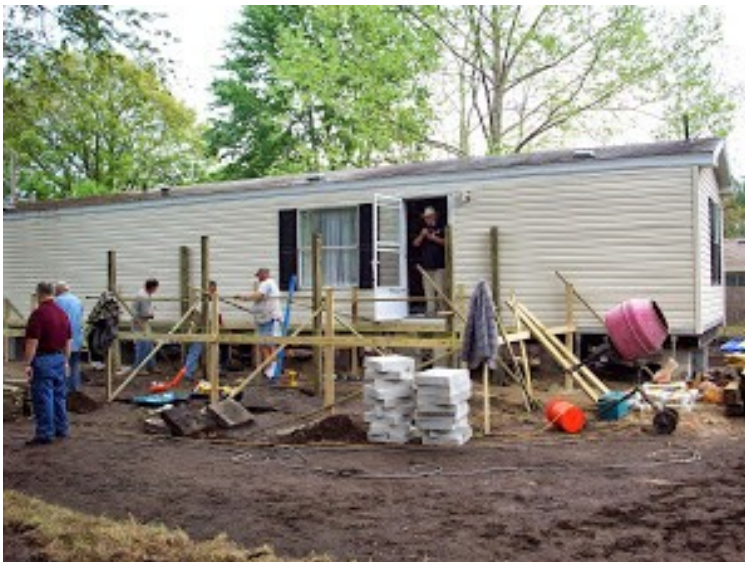
Church men build a new deck and wheelchair ramp
